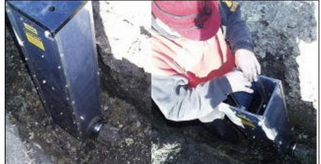
Fig 4. Installation of a water control structure. At left, inflow and outflow pipes are visible at the bottom of the structure. At right, one of the baffles that are used to set water height, is removed.
