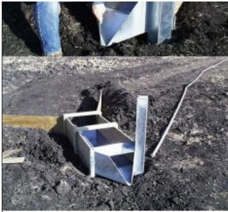
Fig 2. One of four newly installed H-flumes for measuring surface runoff. Berms can be seen extending away from the wing-walls of the flume. Above, BAE Masters student, Gary Feyereisen, works on installation of the flume.
