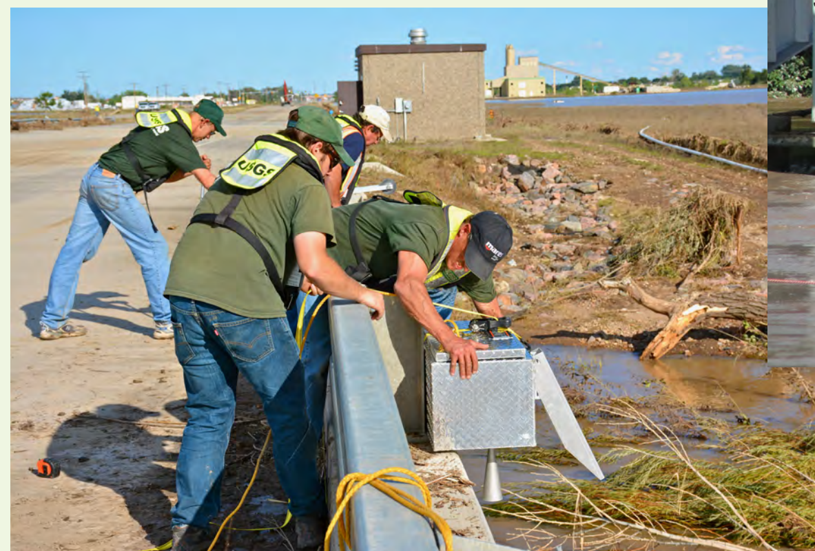
Installation on a bridge with a damaged streamgage
