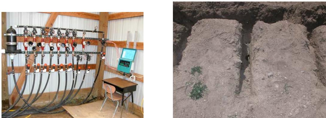
Figure 2 – Computer and valve controls for the SDI research site and open trenches for SDI lines.
