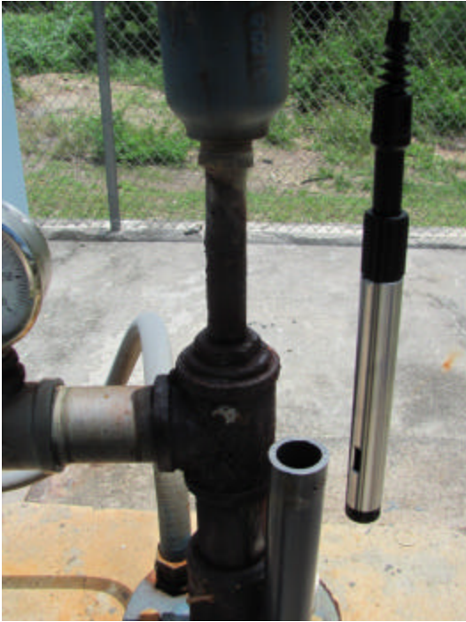
Figure 6: installing probe in IF-205
