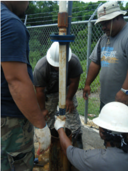
Figure 4: lowering drop pipe, sounding tube, well cap
