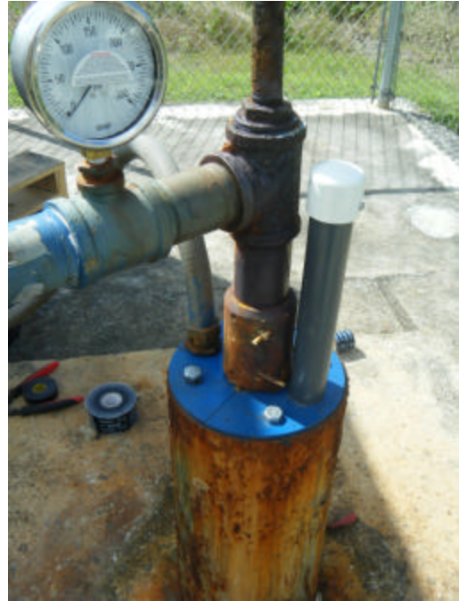
Figure 5: new well cap and sounding tube
