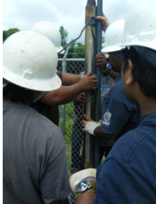
Figure 3: installing sounding tube
