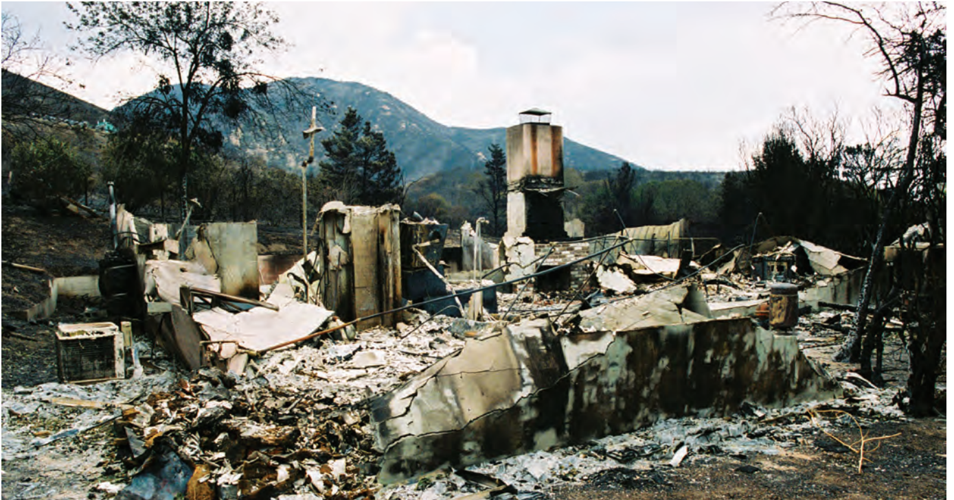
A wildfire left very little of this home near San Bernadino, California, in October 2003. FEMA photograph by Kevin Galvin.
