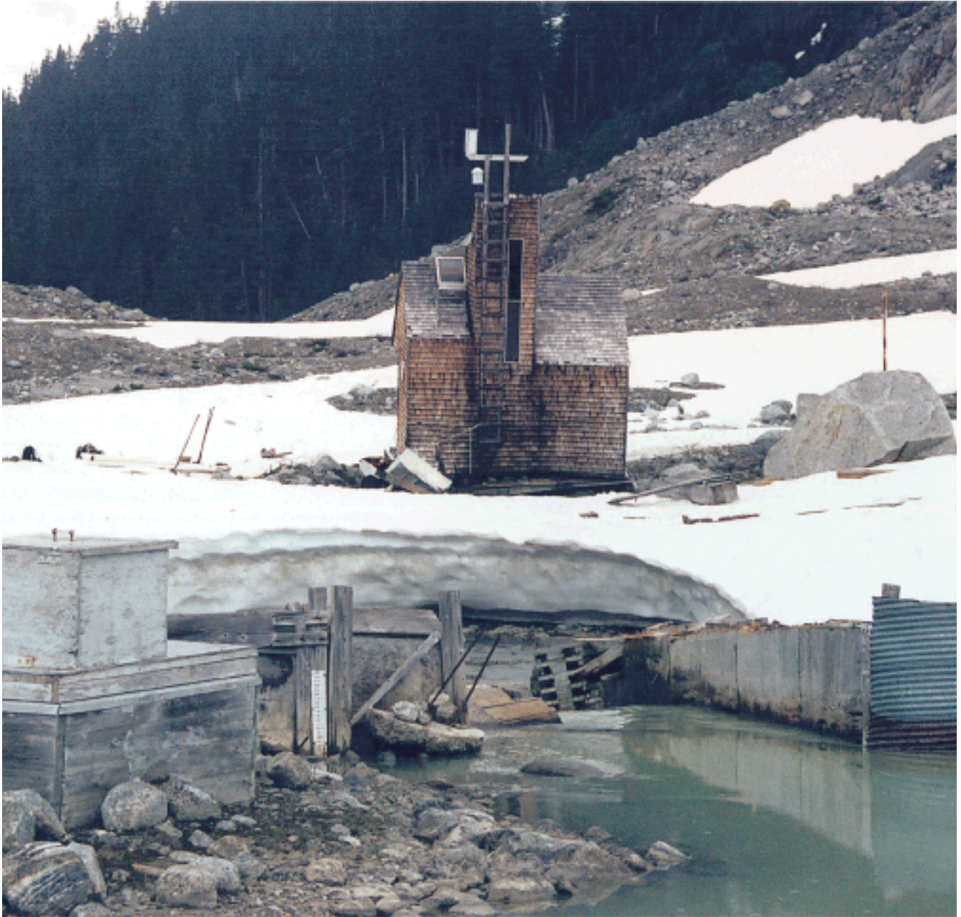
Figure 22. South Fork Cascade River gage house after it was hit by an avalanche.
