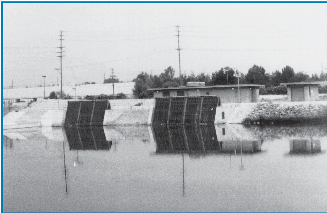
B. Diversion downstream from Imperial Highway, looking across from left bank [flow is to the left] (November 7, 1996, streamflow is approximately 190 cubic feet per second).
