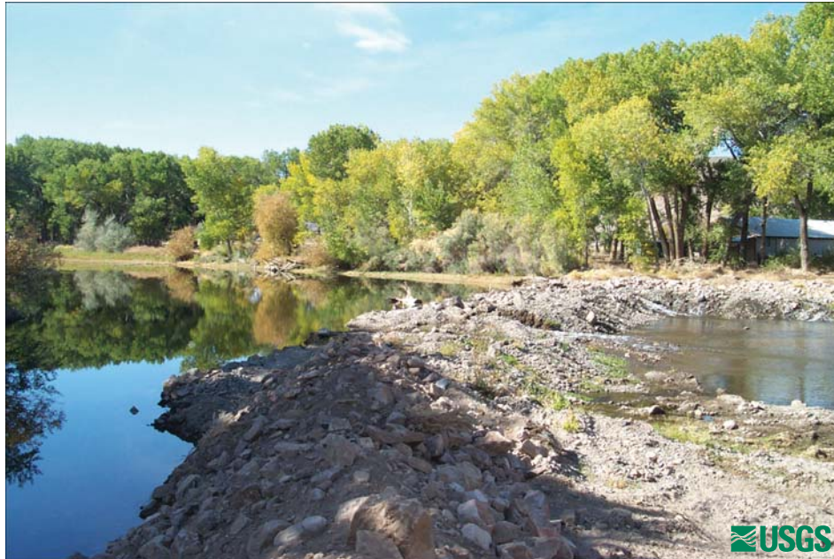
Figure 7. Typical low-head dam along Carson River.
