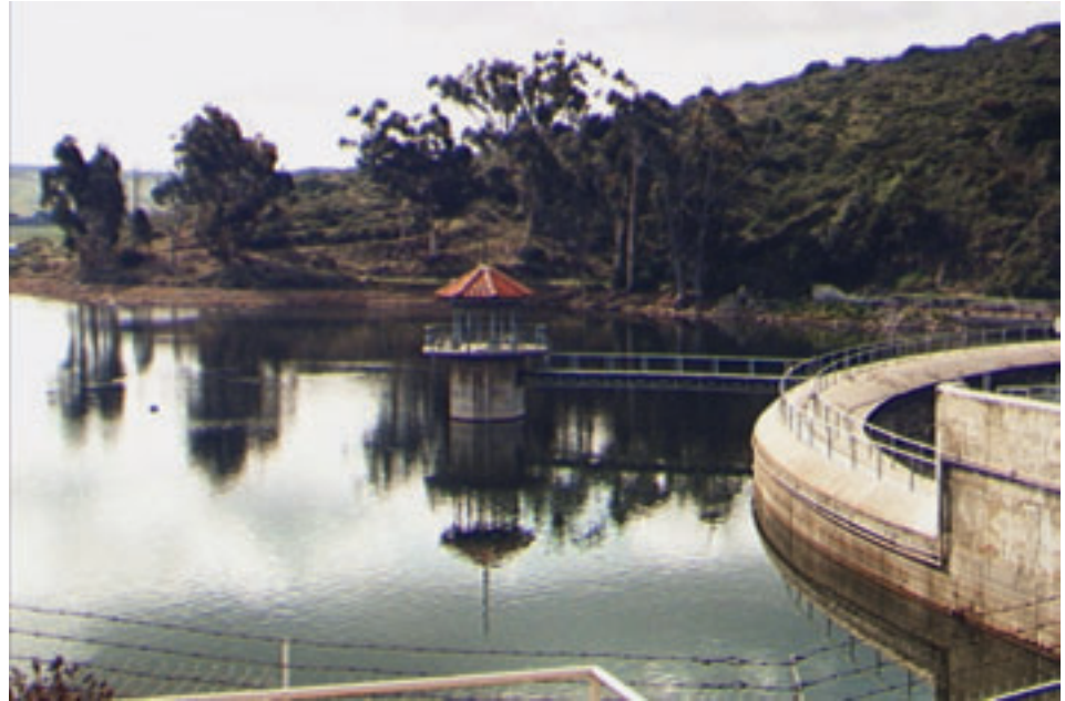
Figure 2. Sweetwater Reservoir, dam, and intake tower for the Sweetwater Authority's Perdue Water Treatment Plant.
