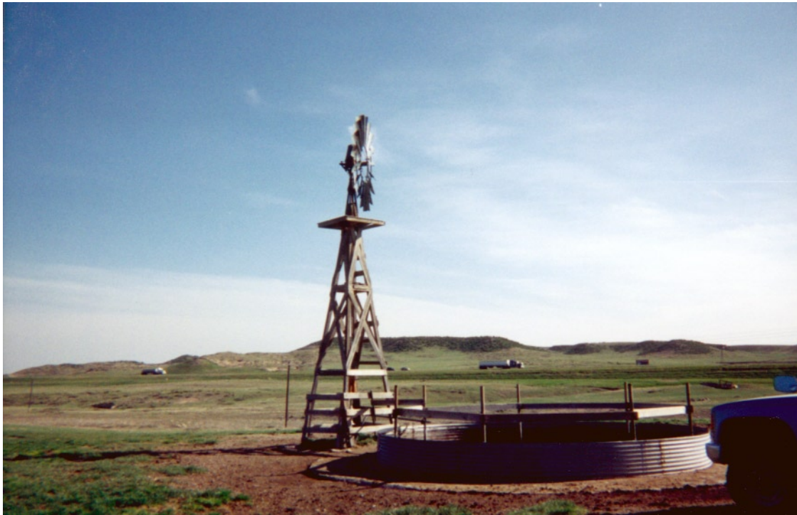
Wind-powered well and livestock watering tank in Platte County, Wyoming (Photograph courtesy of J.P. Mason, U.S. Geological Survey.)
