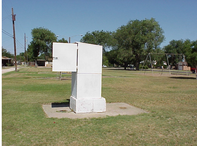
Observation well equipped to measure ground-water levels continually in Lea County, New Mexico (Photograph courtesy of R.R.Cruz, U.S. Geological Survey.)
