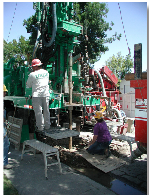
Figure 3. Drilling a monitoring well in Modesto, California.
