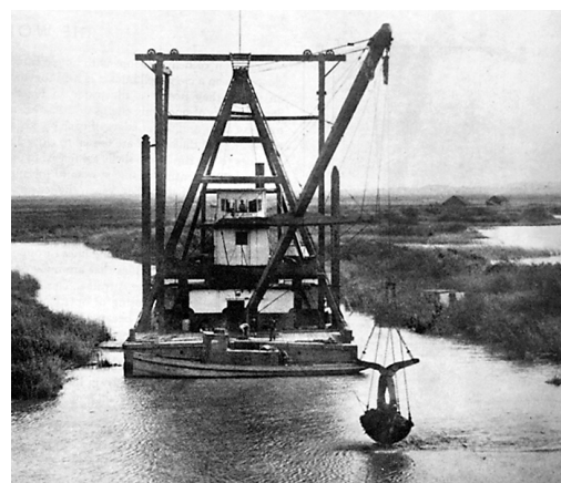
A clamshell dredge operates near Sherman Island, ca. 1907.
