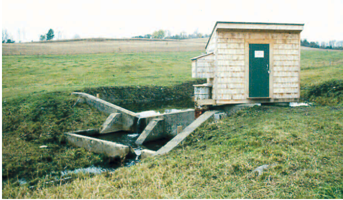
This streamflow-gaging station (W-2) records streamflow from a 59-hectare agricultural catchment. The USGS operates 4 of the original 17 Sleepers River streamgages, as well as 5 new gages on small streams within the forested headwater catchment W-9.
