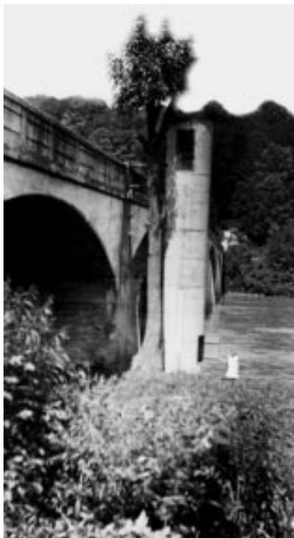
Figure 1. Streamflow-gaging station in nearly continuous operation since 1895 on the French Broad River at Asheville.
