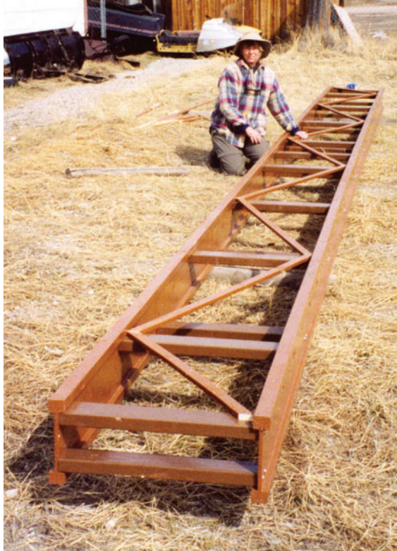
Figure 32 —Close up of the footbridge used at Half-moon Creek without decking (to show construction).
