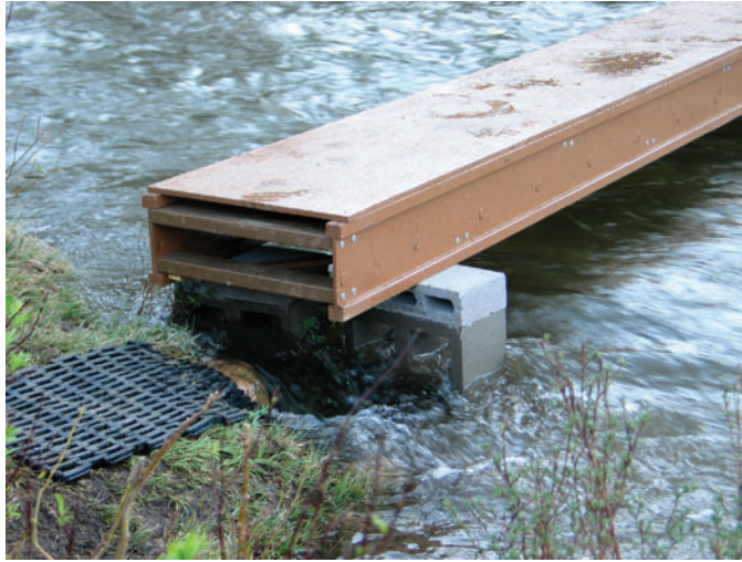
Figure 21 —Foot mats placed at the end of a footbridge to protect the grass from trampling and to avoid creating a mud puddle.
